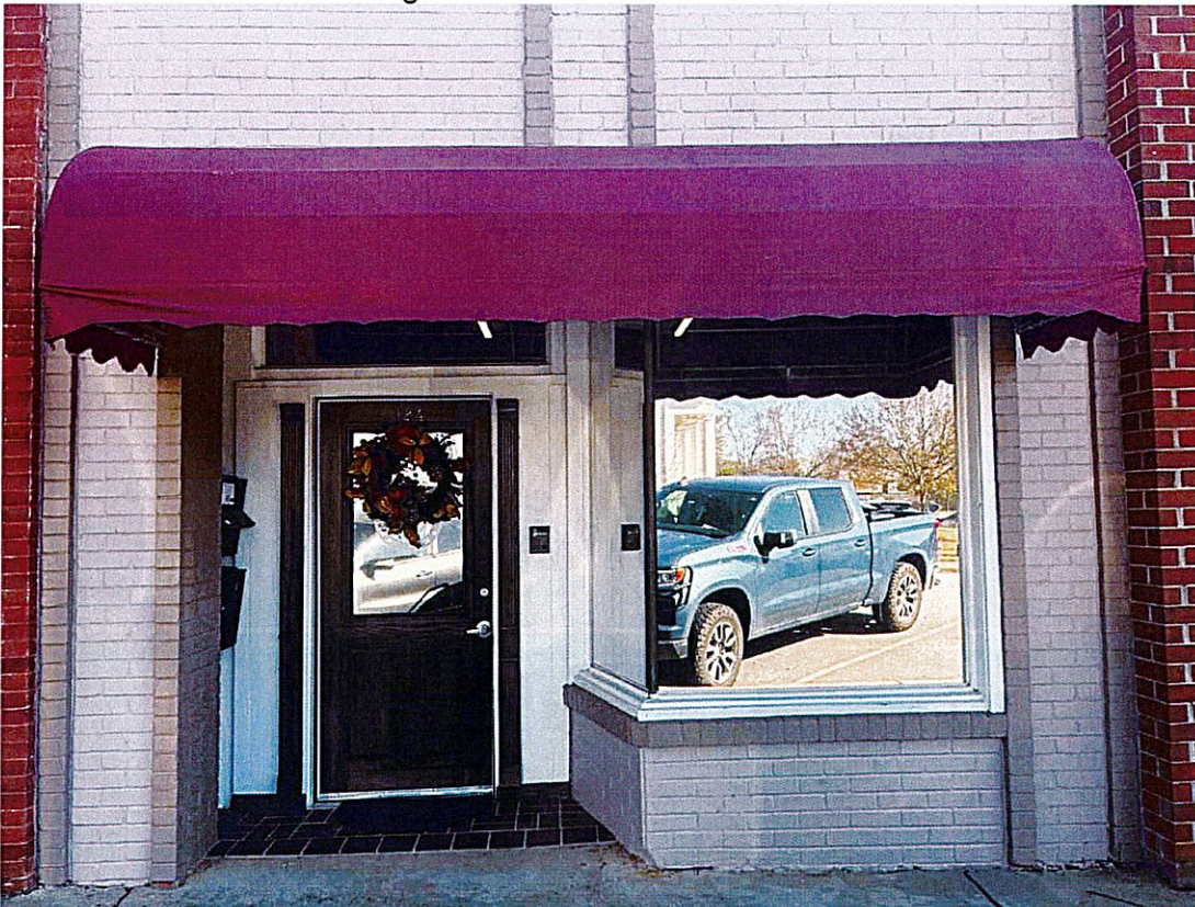
124 Exchange Street. Image sent to Staff on 12/12/2025 showing the installed reflective tinted mirrors.
