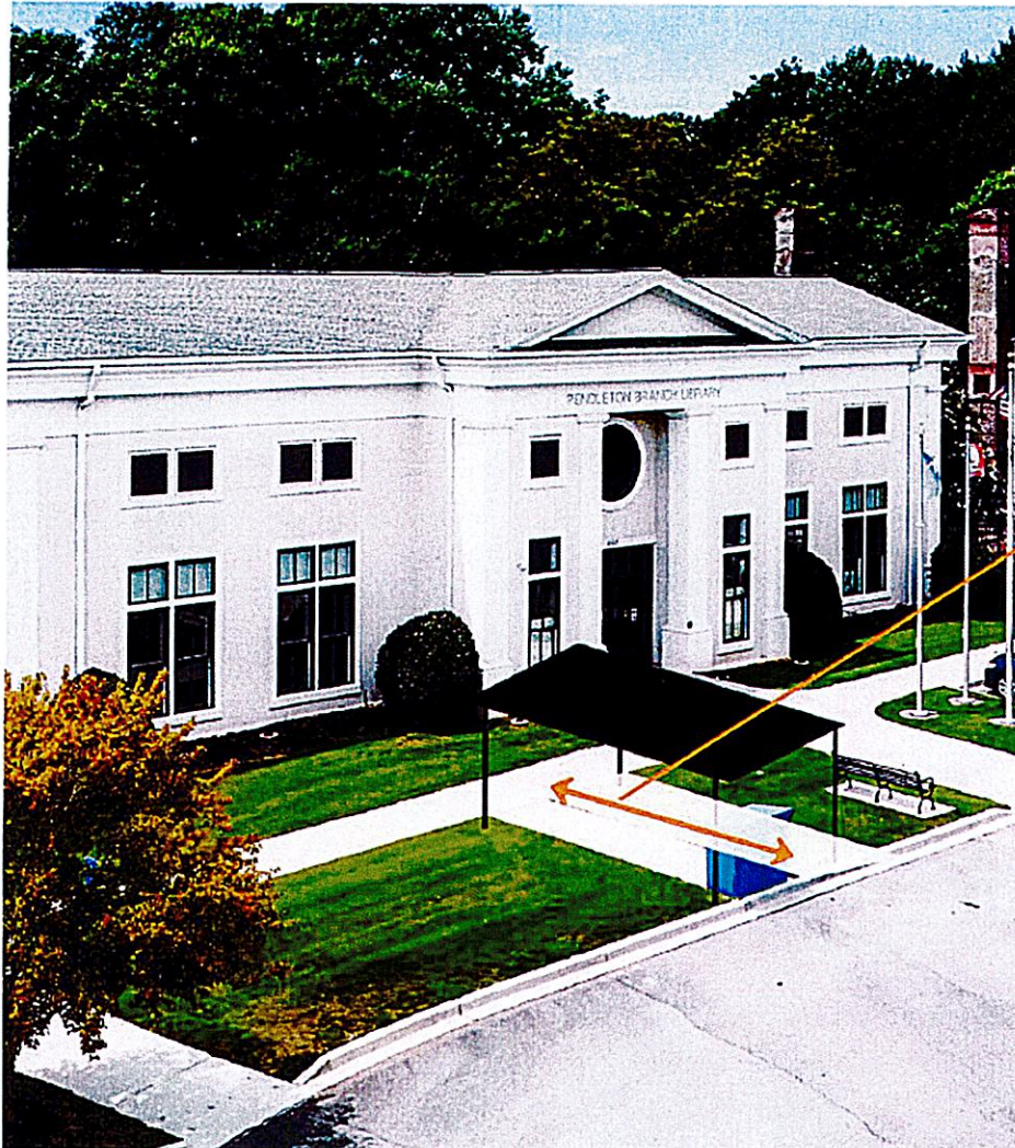
Accessory structure approved by BOZA on December 9, 2025. Locker design included in staff report attachments.
