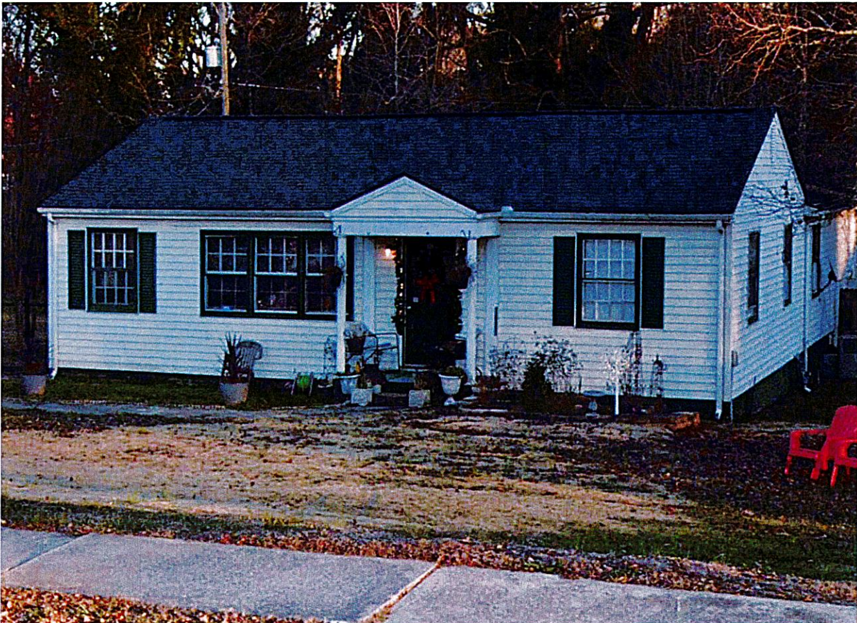
842 Greenville Street, Image Taken From Google Dated December, 2025
