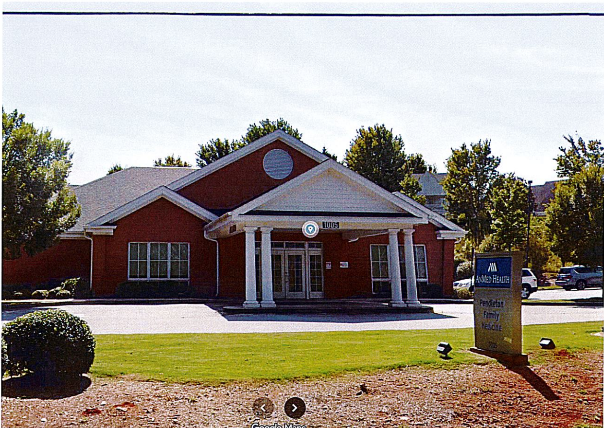
124 Exchange Street. Image sent to Staff on 12/12/2025 showing the installed reflective tinted mirrors.
